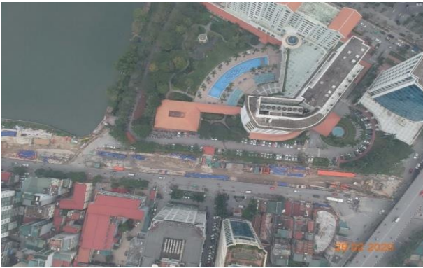
Fig. 5 – Construction site of ramp and surrounding buildings
