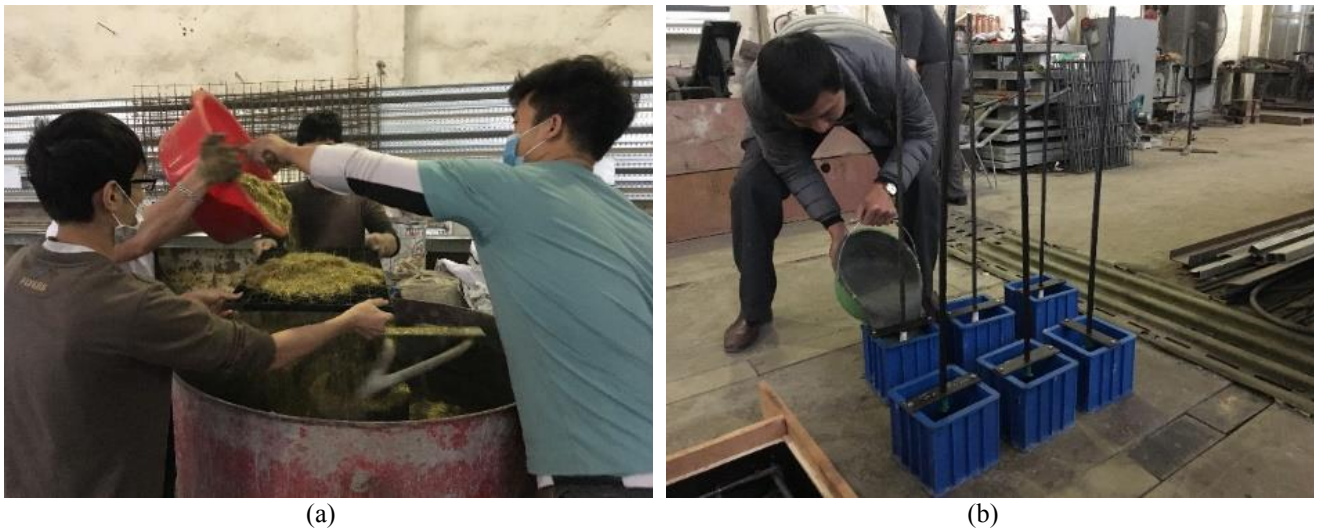
Fig. 1 - (a) Mixing and (b) placing of UHPC mixtures
