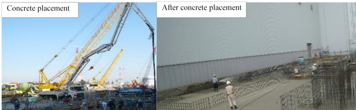
Fig. 11 – Construction status using recycled aggregate concrete [46].
