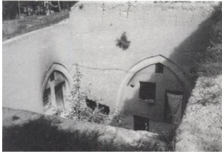
Figure 1. The type of loess cave dwelling at Xian, China that collapsed in great numbers during the 1956 Great Shanxi earthquake (Krinitzsky et al., 1993).
