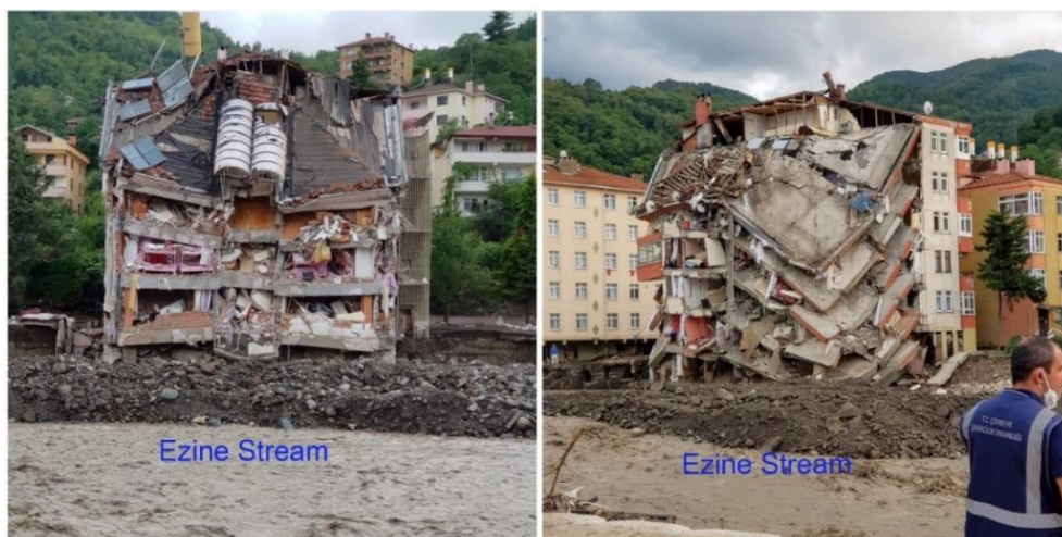
Figure 6: Many buildings located on the edge of the Ezine Stream were destroyed in Bozkurt flood (Photos: Vedat Avcı)
