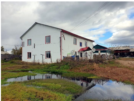
Fig. 16. “Orphanage” in the Yunkyr village, September 2022. Photo by A.A. Suleymanov.
