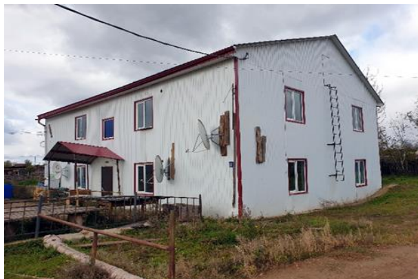
Fig. 17. “Orphanage” in the Yunkyr village, September 2022. Photo by A.A. Suleymanov.
