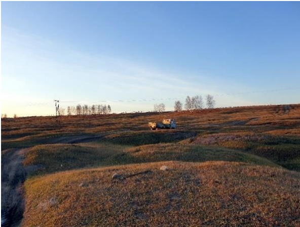
Fig. 32. Examples of deformation of intra-village communication routes in the Yunkyur village, September 2021. Photo by A.A. Suleymanov.
