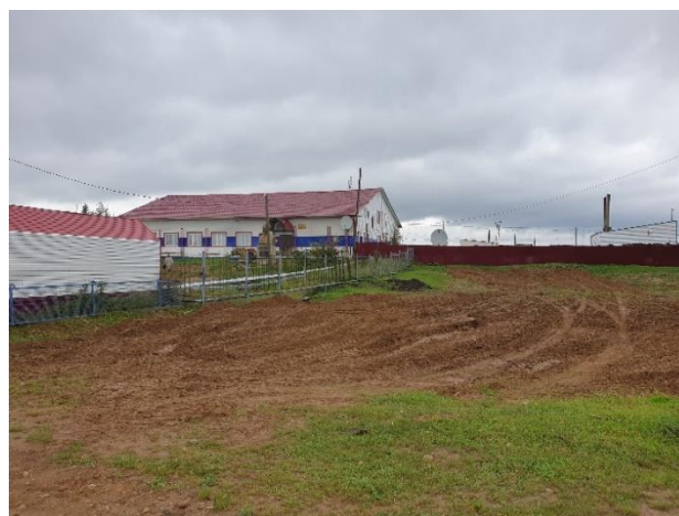
Fig. 43. Backfilling of the area around the club to reduce the activity of thermokarst processes, Yunkyr, September 2022. Photo by A.A. Suleymanov.
