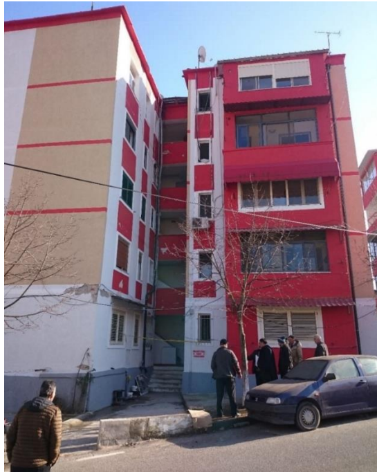
Fig. 22 The examined building
