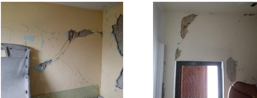
Fig. 23 Typical damage patterns observed at several locations of the studied template design
