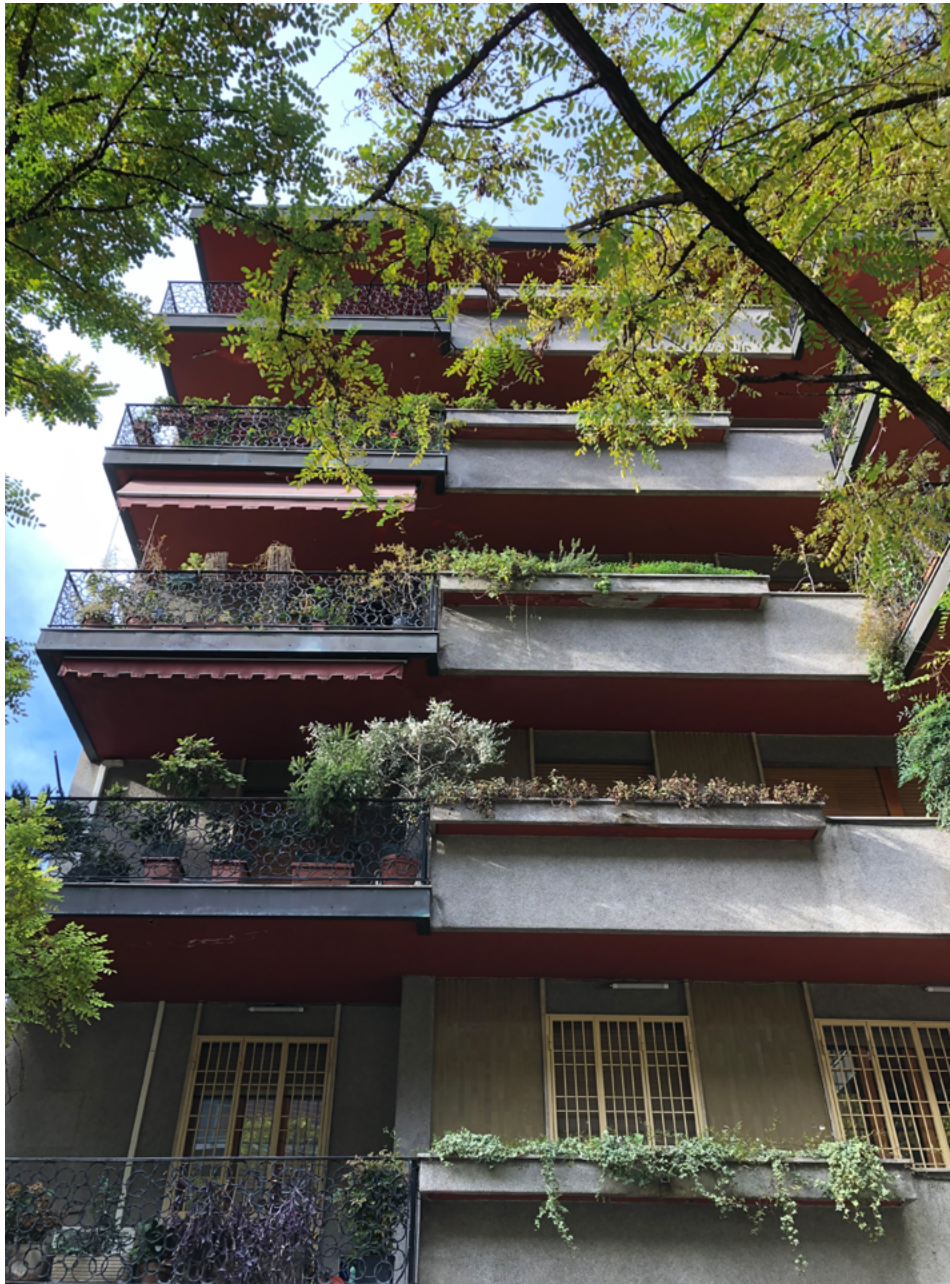
Figure 2. Deep balconies in residential building in Milan. (Photo: António Carvalho, 2023).
