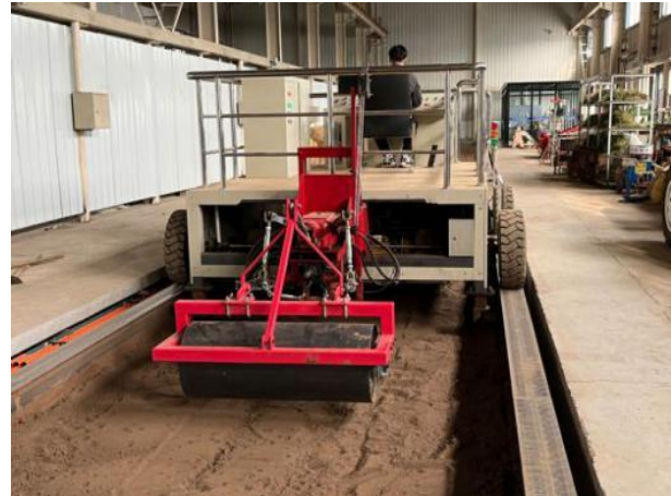
Fig. 12 - Flatten out the land
