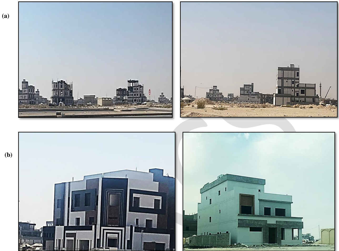
Fig 2:- (a) Incomplete homes in Al Mutlaa City and (b) Completed homes in Al Mutlaa City (Photos taken by Iphone 11 pro max, Author 2022)
