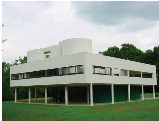
Figure 2. Villa Savoye, Le Corbusier. Poissy-sur-Seine, France, 1929-1931. Main façade. Photo : Valueyou (talk). https://en.wikipedia.org/wiki/File:VillaSavoye.jpg
