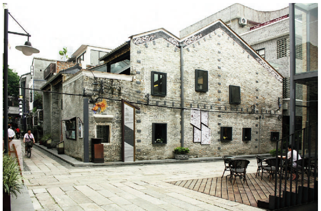
Fig. 12 | Project of conservation and restoration of the existing building (credit: Liu et alii, 2016).
