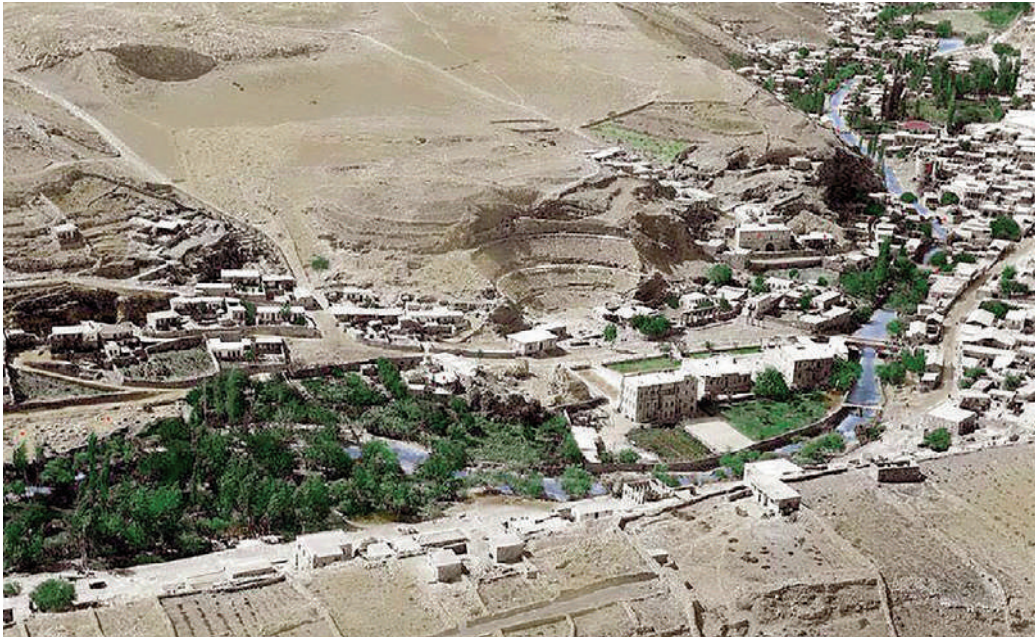
Fig. 1 | An aerial view of the Seil of Amman in 1932 looking over the downtown and towards Ras al-Ein on the upper right (credit: American Colony, Photo Department, Photographer, 1932).
