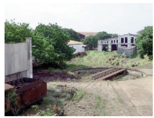
Fig. 10 | Togorail buildings built-in 1911 awaiting conversion (credit: P. Thépot, 2020).
