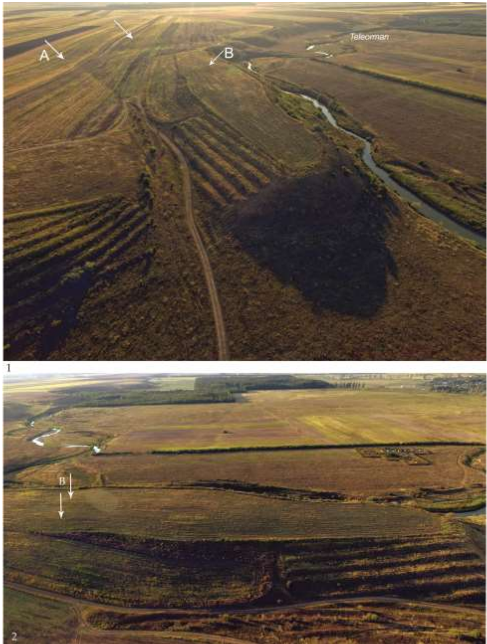
Fig. 22. Orbeasca de Sus–Cetate site, aerial views: 1. From east; 2. From south; A and B label the two observed fortification lines.
