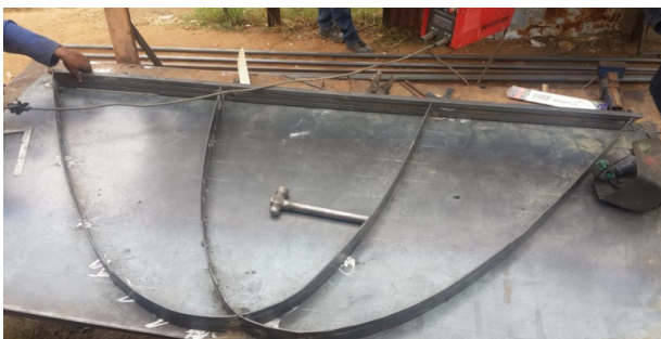
Fig.8. The modified CPC being constructed
