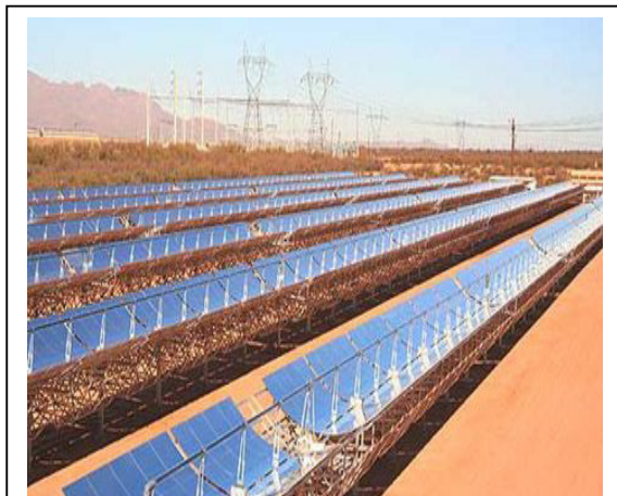
Fig. 5. Solar field comprising of parabolic trough shaped mirrors arranged on rows.
