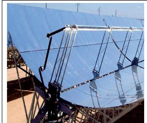
Fig. 4. A typical parabolic trough-mirror.
