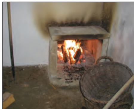
Figure 25. Reconstructed praefurnium of a functioning underfloor-heating system (2006). (Franz Humer, Haslau a. d. Donau).
