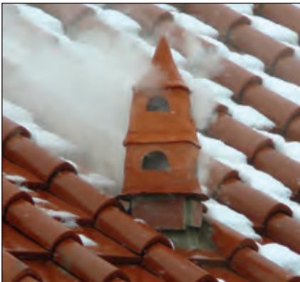
Figure 19. Roof with reconstructed tiles and functioning chimney (2007). (Franz Humer, Haslau a. d. Donau).
