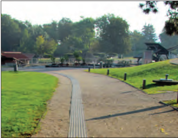
Figure 39. Tactile ground guidance system for the blind (2015). Franz Humer, Haslau a. d. Donau.
