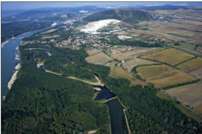
Figure 3. View to Porta Hungarica: River Danube with its wetlands and the bridge in Bad Deutsch-Altenburg. In the far background the city of Bratislava/SK (2003). (Franz Humer, Haslau a. d. Donau).
