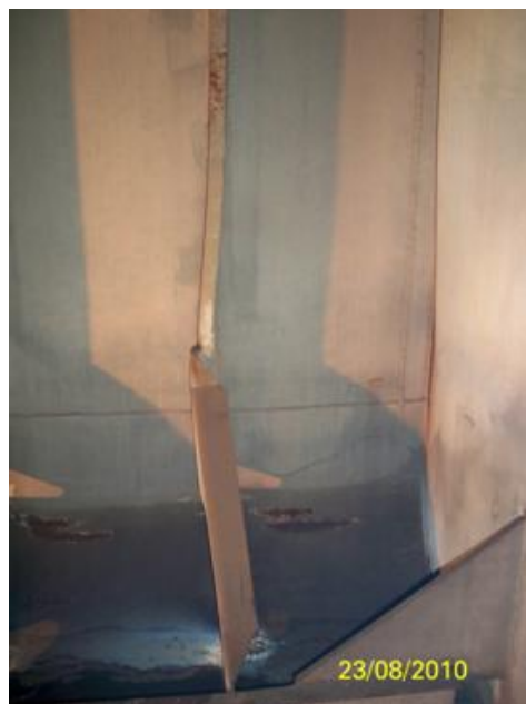
Figure 3. Deformation of the blade in the shell and bottom of the ship
