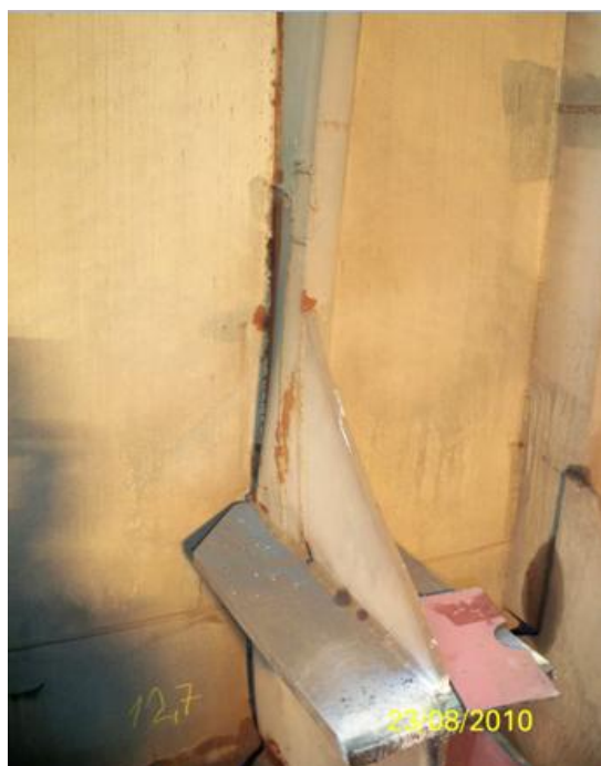
Figure 4. Cutting and removing the portions damaged in a varanga - heart and payment
