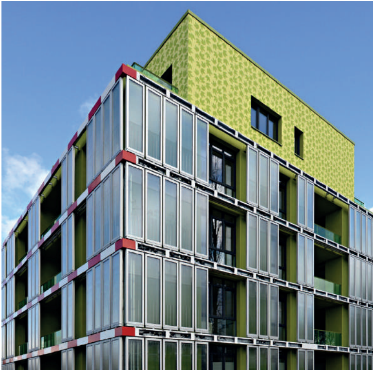
Fig. 7 | BIQ House by ARUP. The south-east and south-west facades are covered with panel photobioreactors (credit: ARUP, 2013).
