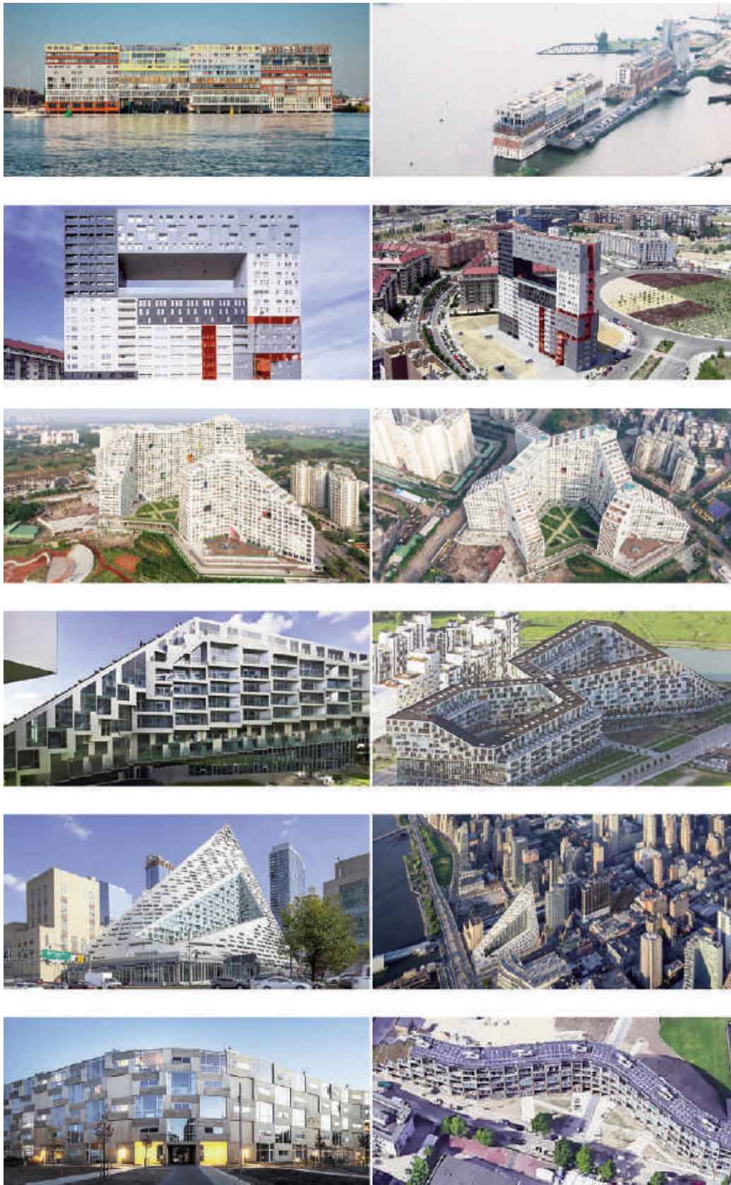
Fig. 5 | The 'containers' of the contemporary in search of content: 'Silodam' in Amsterdam by MVRDV, 2003; 'Mirador' in San-chinarro by MVRDV, 2005; 'Future Towers' in Pune by MVRDV, 2018; '8 House' in Copenhagen by Bjarke Ingels Group, 2006; 'Via 57 West' in New York by Bjarke Ingels Group, 2016; 'Dortheavej Residence' in Copenhagen by Bjarke Ingels Group, 2018 (credits: MVRDV, Ossip van Duivenbode, Jens Lindhe, Iwan Baan, Danica O. Kus, Iwan Baan, Rasmus Hjortshøj).
