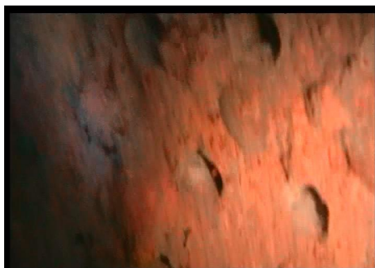
Figure 2. The process of clogging in the filter section of the inlet water well is shown.
