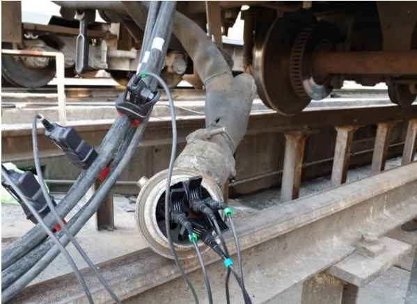
Figure. 8 (a) electric coupler view and (b) measurements taken from the electric coupler
