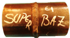
Figure 1. Welded joint welding E1
