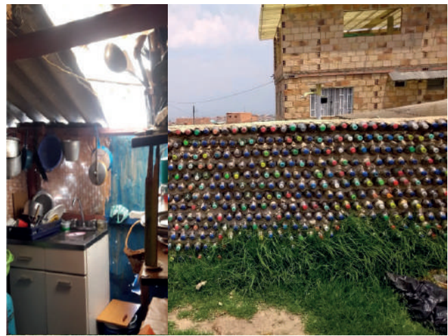
Figure 5. Light litre and Community room wall [18].
