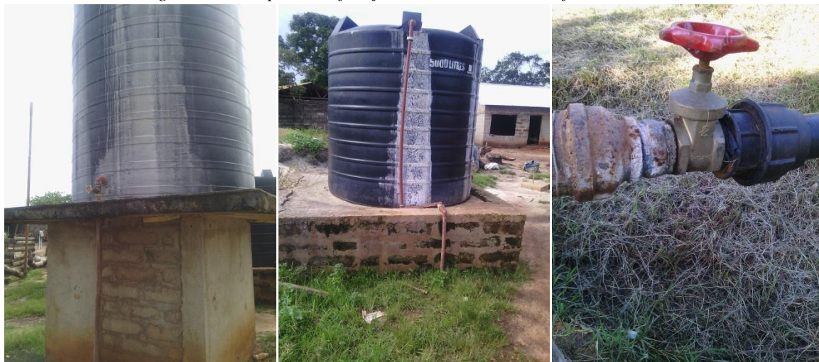
Plate 4.2: Whitish strips formed due to presence of Calcium in water at Pangani
