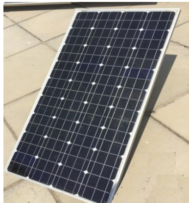
Figure 10: Solar panel fixed on building roof with 30° inclination, without tracker system
