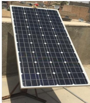
Figure 12: Solar panel equipped with a double axis tracker
