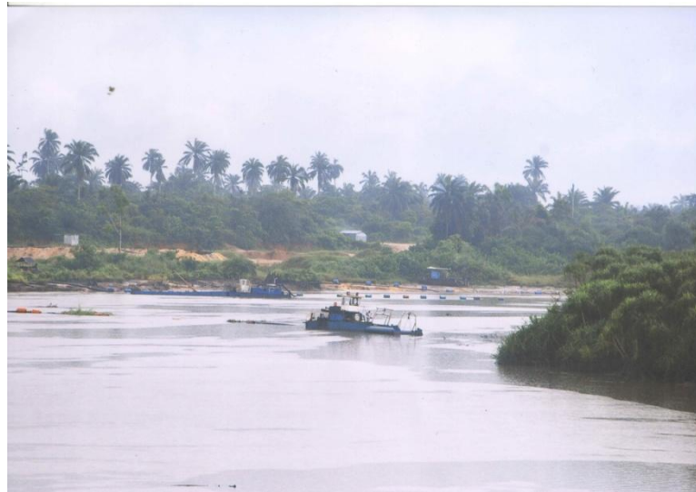
Figure 2: A typical Dredging Fleet
