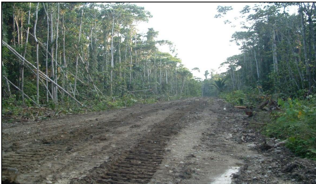
Figure 1: Condition of Road in Research Location before Construction
