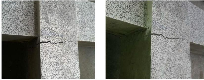
Figure 11. Cracking under concrete beams. Source: [1]
