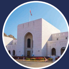
Heating, Ventilation & Air Conditioning (HVAC) and Building Management Systems
