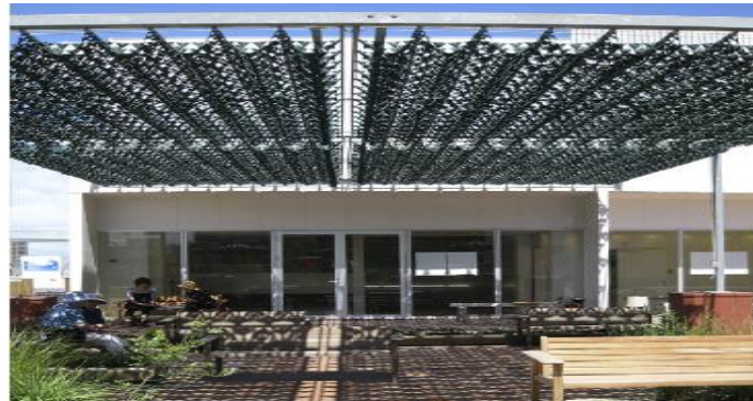
Figure 5: Fabric fractal sunshade at the roof garden of a shopping centre in Kagoshima, Japan [24]
