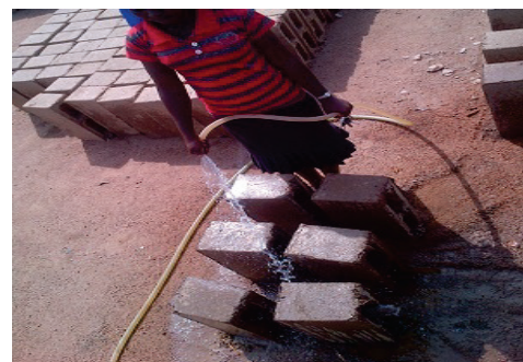
Fig 9: Curing of sandcrete blocks
