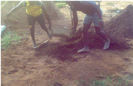
Fig 4: Manual method of producing sandcrete blocks
