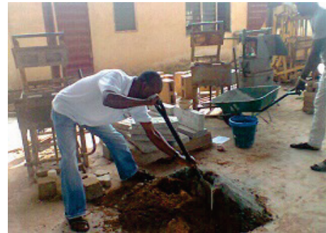
Fig 5: Mixing of cement-sand mortar prior hand ramming method of production
