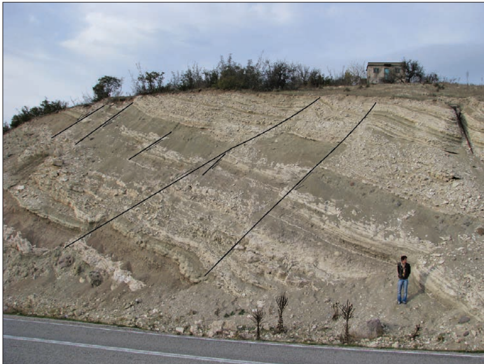
Figure 11- Syn-sedimentary normal faults affecting the claystone, marl, limestone and tuff layers.
