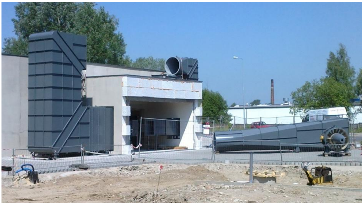
Figure 1. Construction of the aerodynamic tunnel and measuring chamber (27.05.2014)
