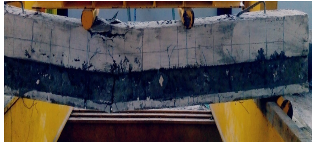
Fig. 24 Crack pattern of beam with web bonded steel plates of 80mm width
