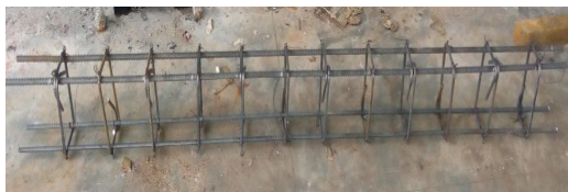
Fig. 2 Reinforcement of control beam
