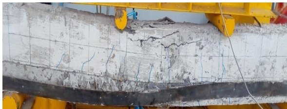
Fig. 18 Crack pattern of beam with web bonded steel plates of 1.6mm thick
