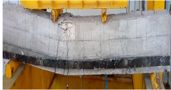
Fig. 23 Crack pattern of beam with web bonded steel plates of 40mm width
