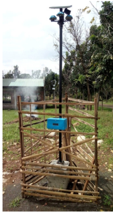
Fig. 5 Installation of Air Quality Monitoring Device for Gaseous and Particle Pollution
