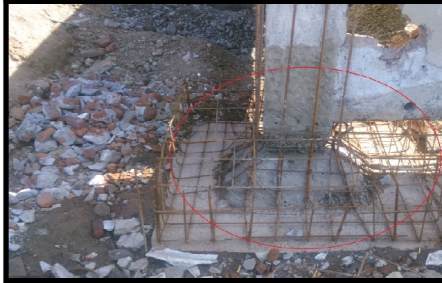
Fig. 8 Shows that footing is strengthen with extra reinforcement
