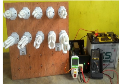
Fig. 3 Testing without load
