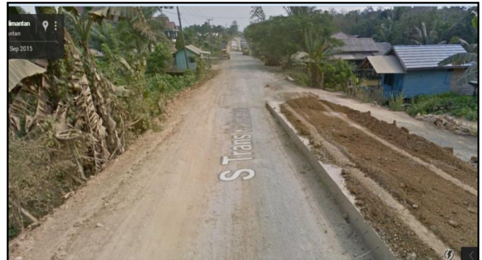
Fig.5. Picture of Project Site
