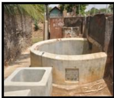
Station IV (Pragasapuram open well)
