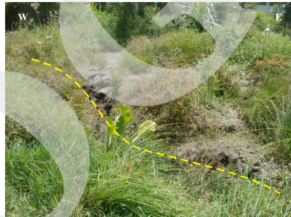
Figure 9. A photograph showing the small pond dried out due to the ground surface rupture at Jamur Ujung Village. The surface rupture track is indicated by a yellow dashed line.
