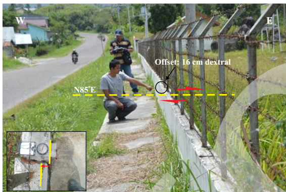
Figure 7. A photograph showing the Site 3 surface rupture continues through a bent brick fence with 16 cm dextral offset. The black circle indicates the centre of deflection of the brick fence. The inset photo shows the lateral offset of the brick fence wall, indicated by a red arrow.
