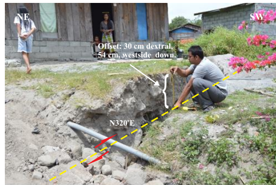
Figure 8. A photograph showing the change of Site 3 surface rupture orientation to 320°, exhibiting 30 cm dextral offset and 54 cm normal offset with west side moving down.
