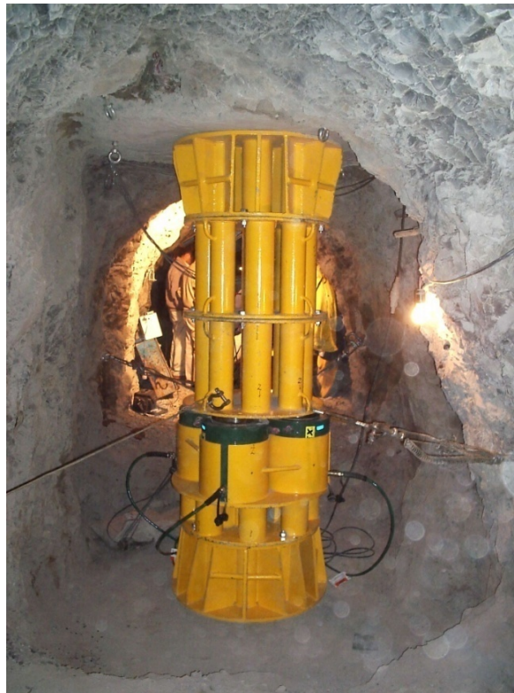
Figure 2. Plate jacking test operation.
