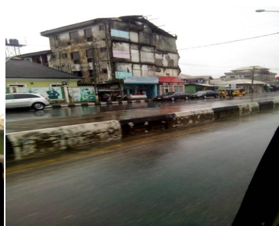
Plate 2A: severed building along Ada George road
