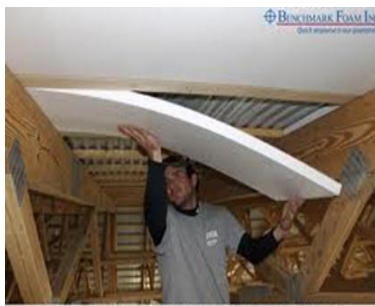
Figure 5: EPS under steel roof as insulation [3]
