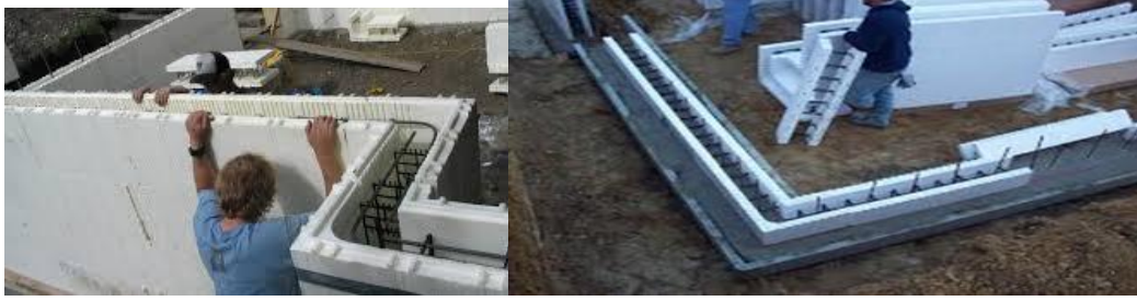
Figure 7: Wall constructed of EPS blocks [3]
