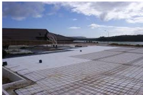
Figure 6: Slab lay of EPS blocks [3]
