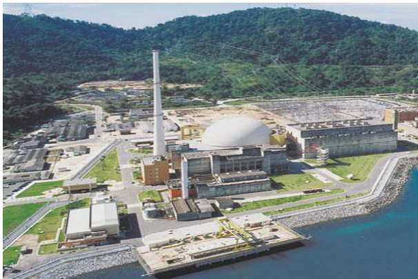
Figure 11: The external formation of Angra nuclear power plant [18].
