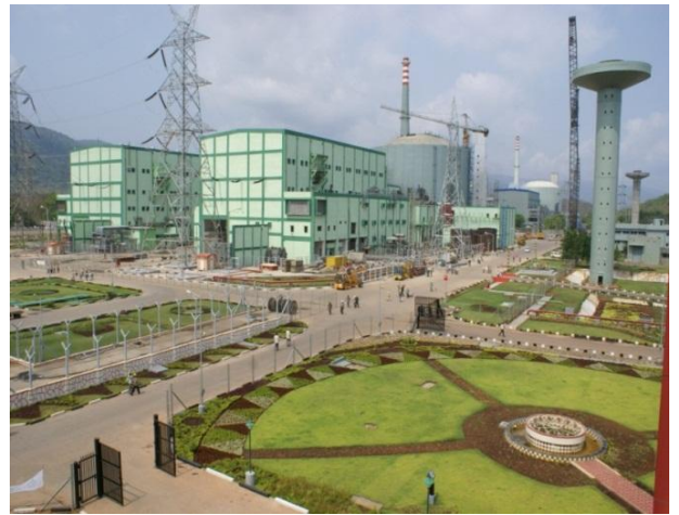
Figure 6: Perspective snapshot of Kaiga nuclear power plant, India [15].
