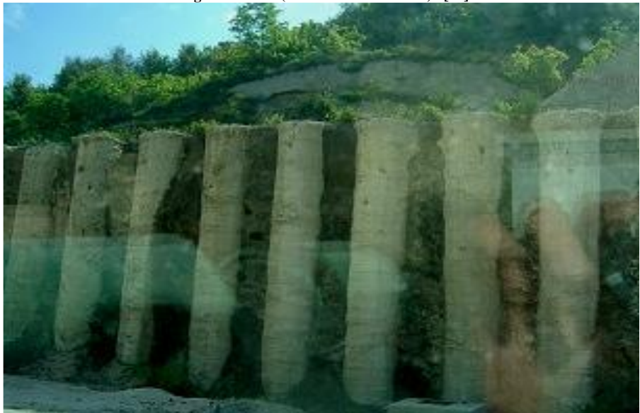
Fig. 15 Pile walls (Source: Marinos 2010). [30]
