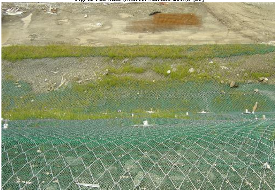
Fig. 16 Embankment with anchors and geosynthetics (Source: Marinos 2010). [30]
