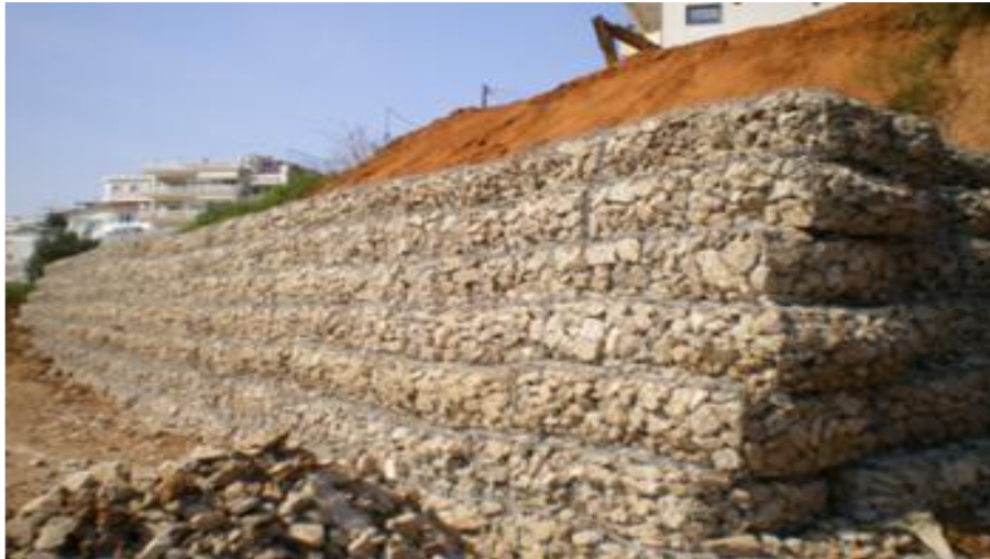
Fig. 18 Retaining wall with gabions (Source: Marinos 2010) [30]
