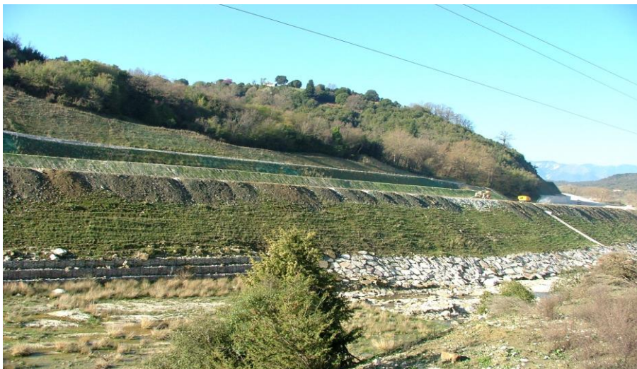
Fig. 20 Slope covered with a special geotextile for vegetation development. (Source: Rozos 2017). [29]
