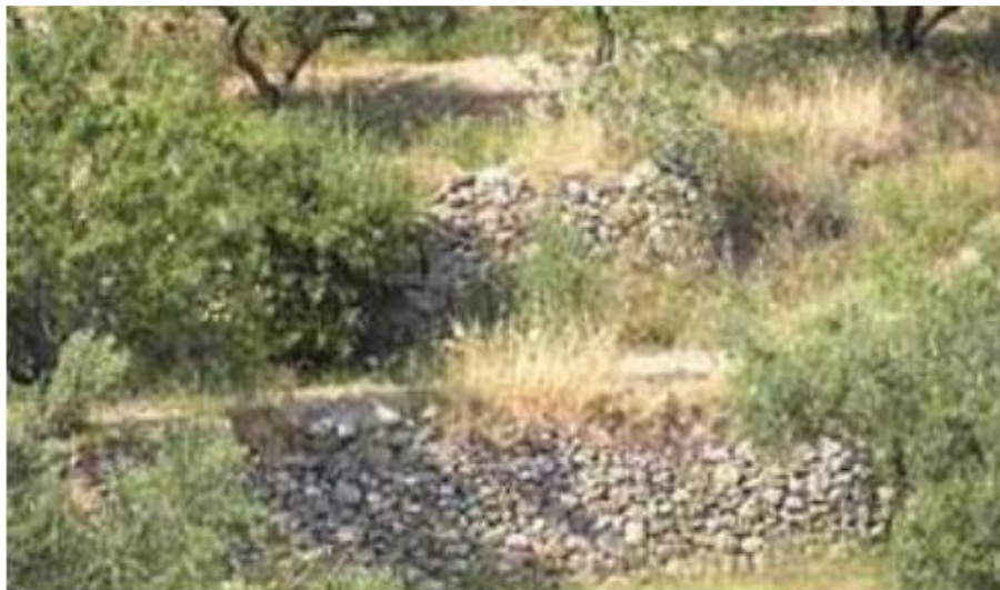
Fig. 17 Drywall retaining wall (Source: Marinos 2010). [30]
