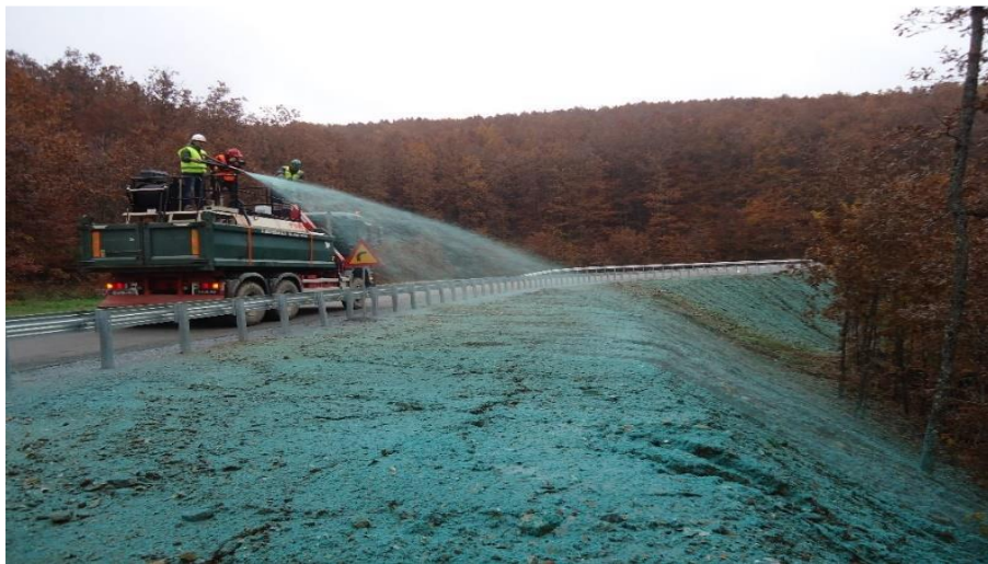
Fig. 25 Hydroseeding in a forest road embankment (Source: Galatsianou 2017). [40]
