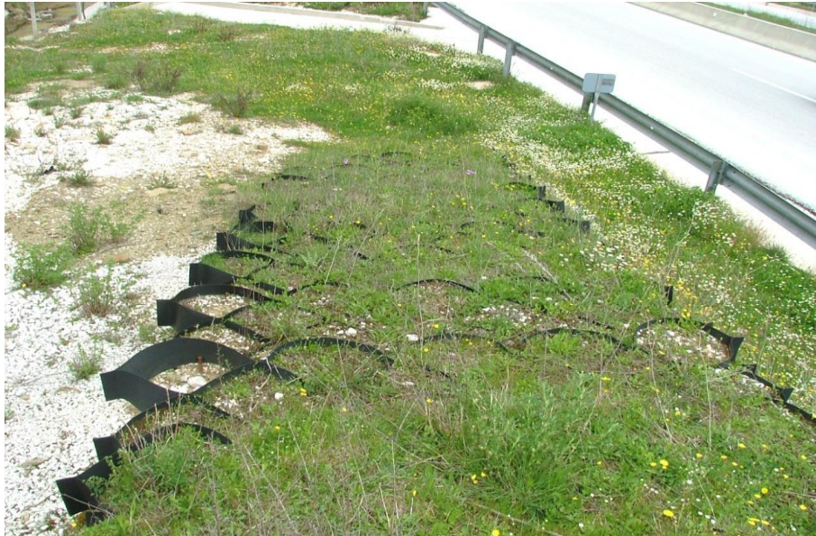
Fig. 21 Polyester geotextile of cellular structure for the growth of vegetation (Source: Rozos 2017) [29]
