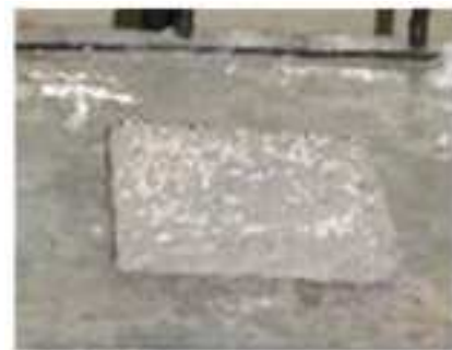
Fig.21 ZPC Tile in Dry Condition
