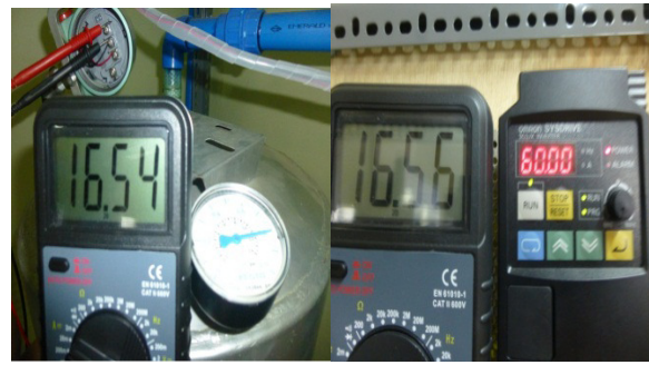
Fig. 3.1: Gathering Test Data using Multi-tester and VFD Display
