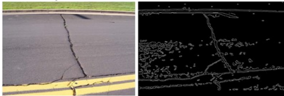
Figure 6: (a) original image. (b) Canny edge detected image
